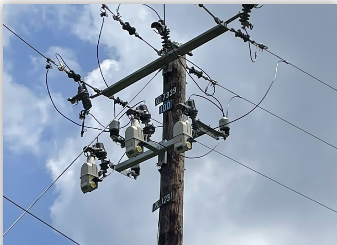
FIGURE 3. The TripSaver II recloser transformed grid reliability for Alabama Power's customers.
