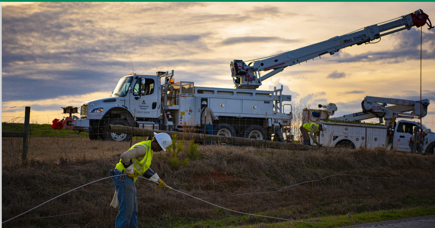
FIGURE 1. Alabama Power crews work to restore power in a rural area.
