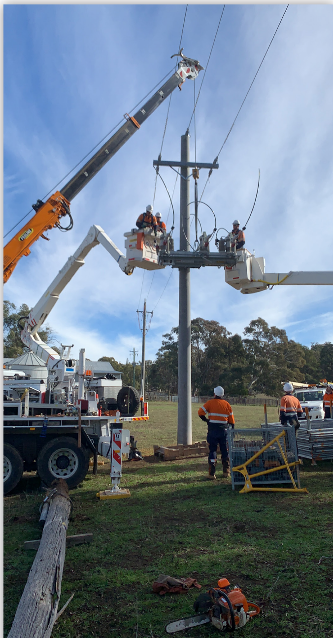
FIGURE 1. Installing an IntelliRupter® fault interrupter with the new high-impedance earth-fault algorithm.
